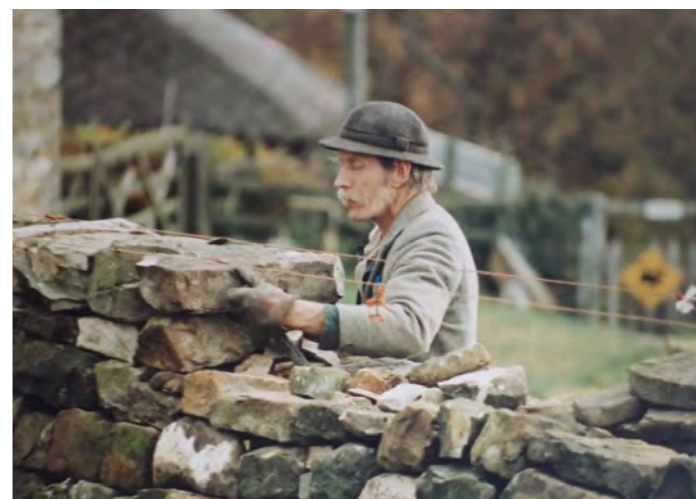
John ensuring his wall is level.
